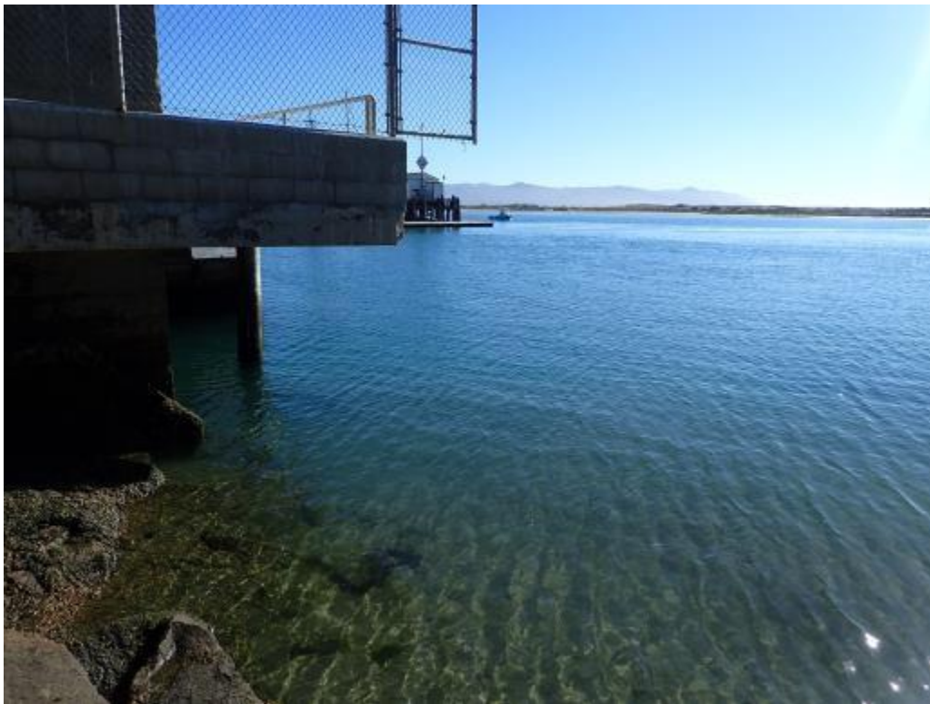
Figure 5 Start of Coleman surveys. Start point is at the edge of the building and extends north 150 m, ending at the elbow in Coleman Beach.
